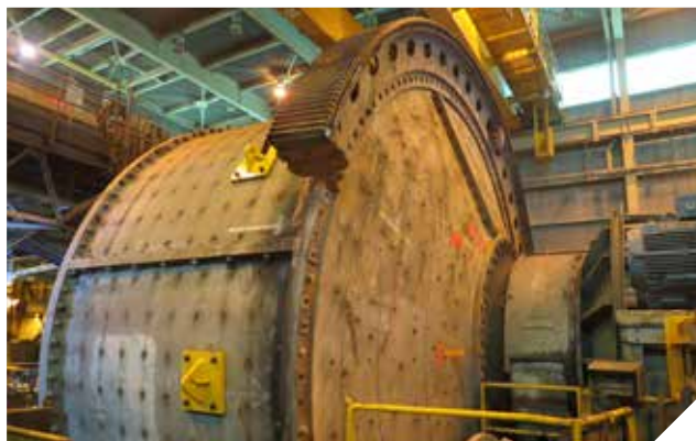
Gear being replaced on an 11,000 HP Sag Mill
