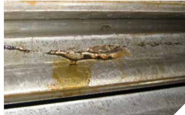
Visual inspection after cleaning uncovered a crack on a gear tooth
