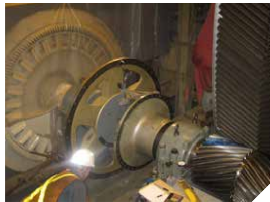
Field personnel align the synchronous motor to the
