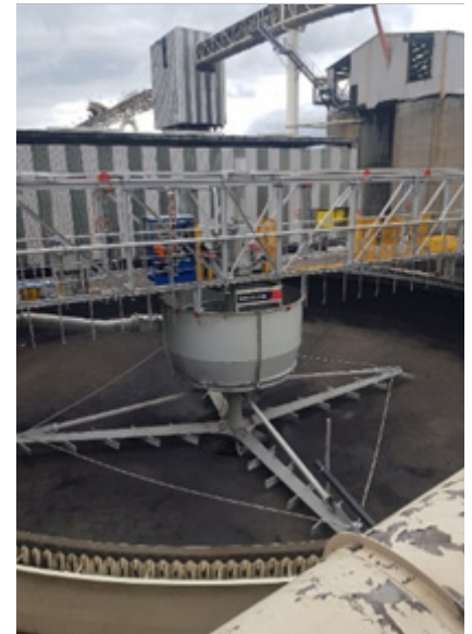
Coal Product Thickener at completion of installation
