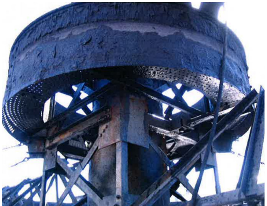
Original thickener feedwell (prior to upgrade)
