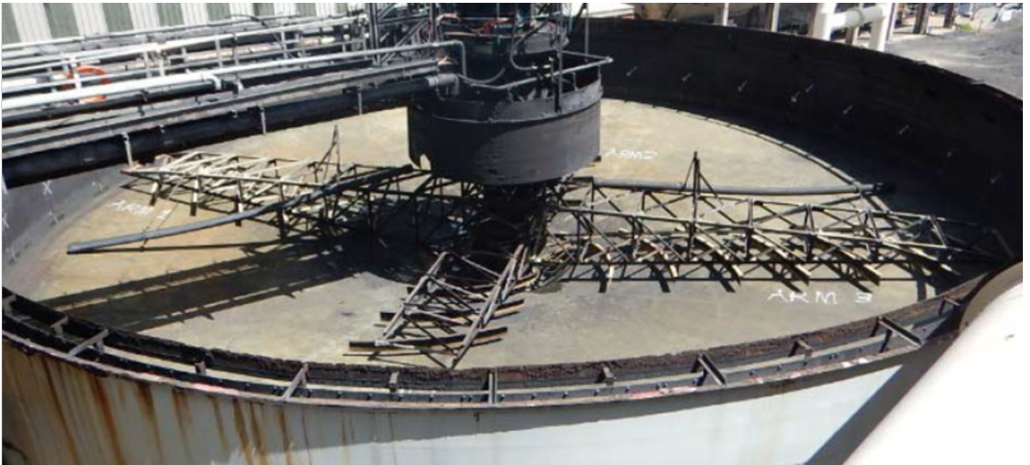
Existing coal product thickener before upgrade (emptied)
